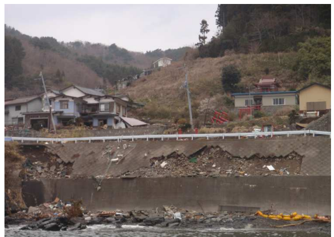
Univ. of Tokyo Tsunami Damage Survey Support
