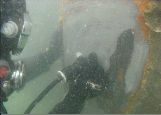
Port Wall Steel Plate Thickness Measuring
